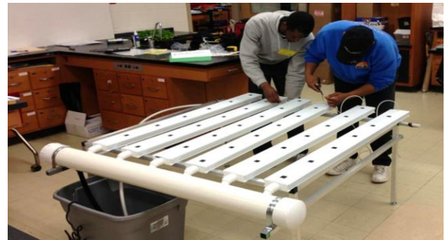
Figure 2. Construction of a small NFT system. (Chris Mullins, Virginia Cooperative Extension)
