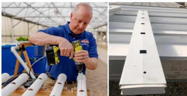
Figure 8. NFT plant channels made from PVC plumbing pipe (left) and prefabricated molded units. (Chris Mullins, Virginia Cooperative Extension)
