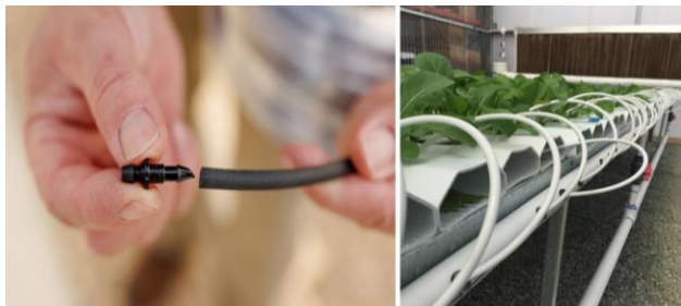
Figure 7. Emitters used in delivery lines of an NFT system. In the left photo, an emitter is being inserted into a black poly tube. In the right photo, emitters are used to connect the white poly tubing to the main manifold at the bottom of the channel support. (Chris Mullins, Virginia State University)
